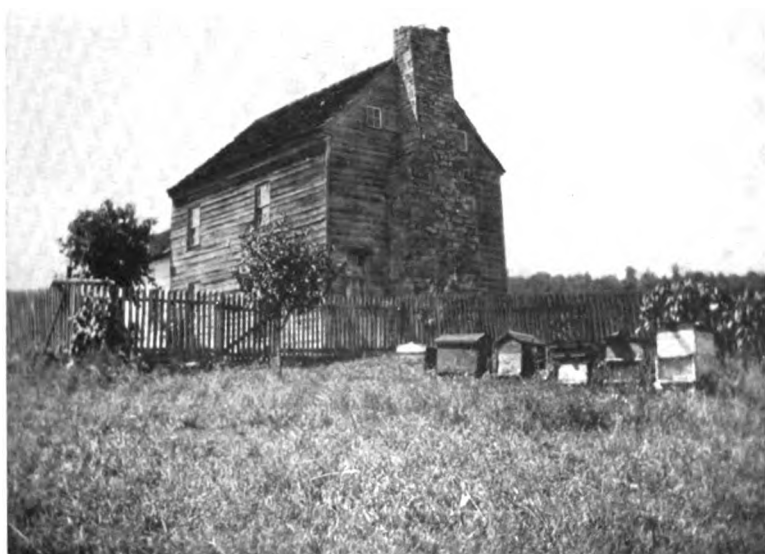
George Paul's original log cabin ; recent addition at the left, all weather boarded.
